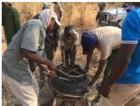
After lunch it was back to the hard work of dropping old telephone poles then cutting and rolling many hundreds of kilometres of the decommissioned telephone wire every day.
