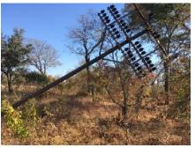
In some areas the rotten & damaged poles are held up by the phone wire alone. If these old poles are NOT carrying any new ADSL or fibre cable, we have been authorised to cut them down so the phone line wires can be easily removed.
